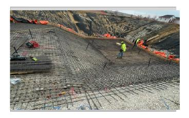
Rebar install @ lap portion of pool floor
